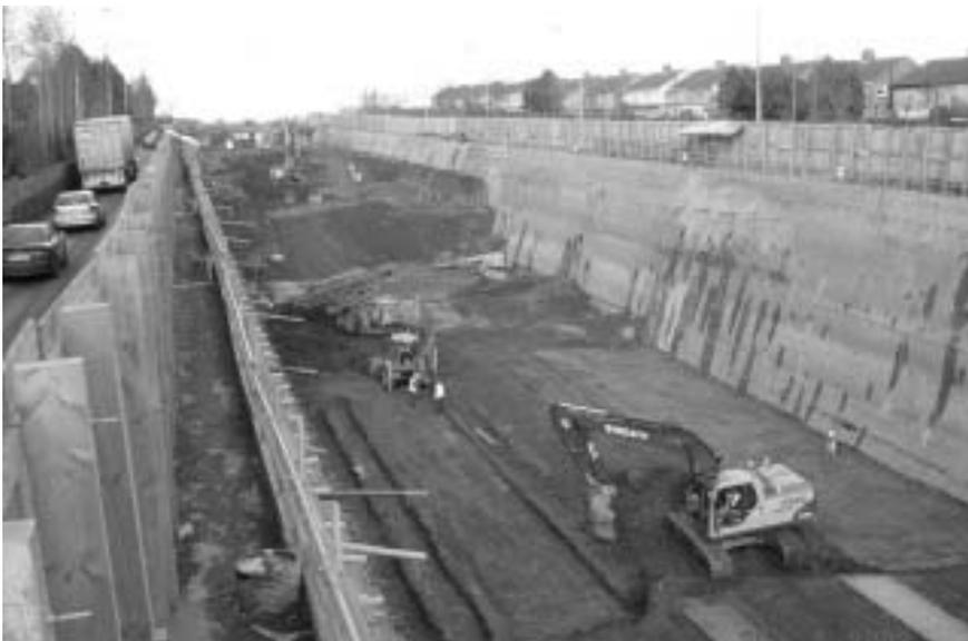
Figure 1. Northern cut and cover section of Dublin Port Tunnel.
